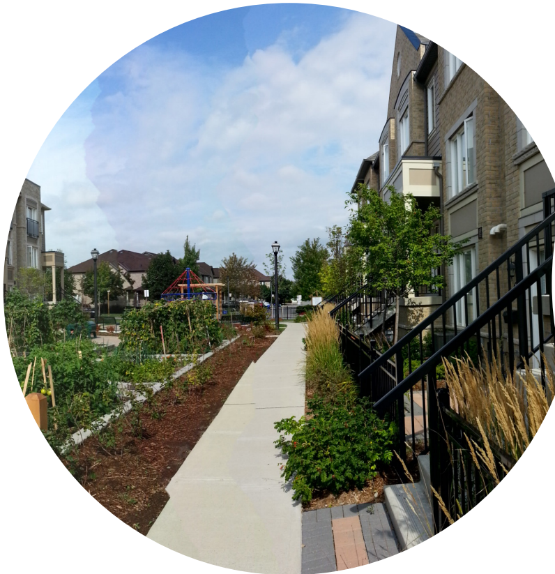
Design standards and zoning provisions that facilitate a variety of housing options and direct development to be more human scaled and pedestrian oriented would make Gravenhurst more all-ages friendly. This award winning development in Mississauga was noted for its compact form, and including a community garden in the shared space between the townhouses.
