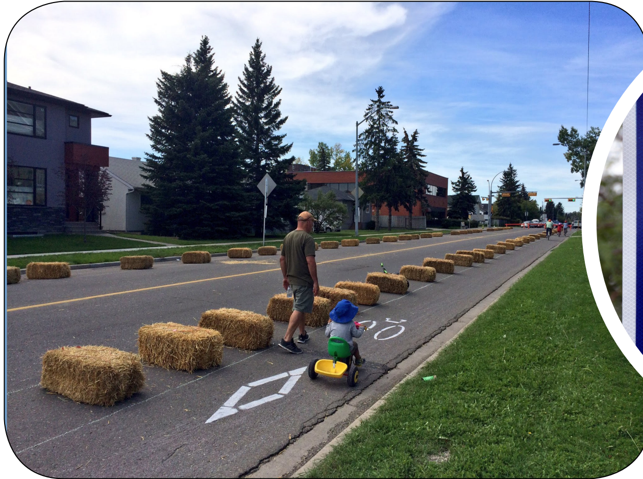
This is an example where temporary urban acupuncture improvements are being used to test out a separated bike lane.
