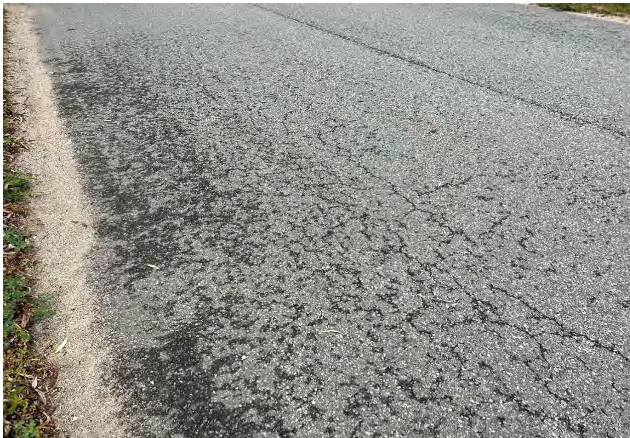
Description of Photo: Alligator crack
