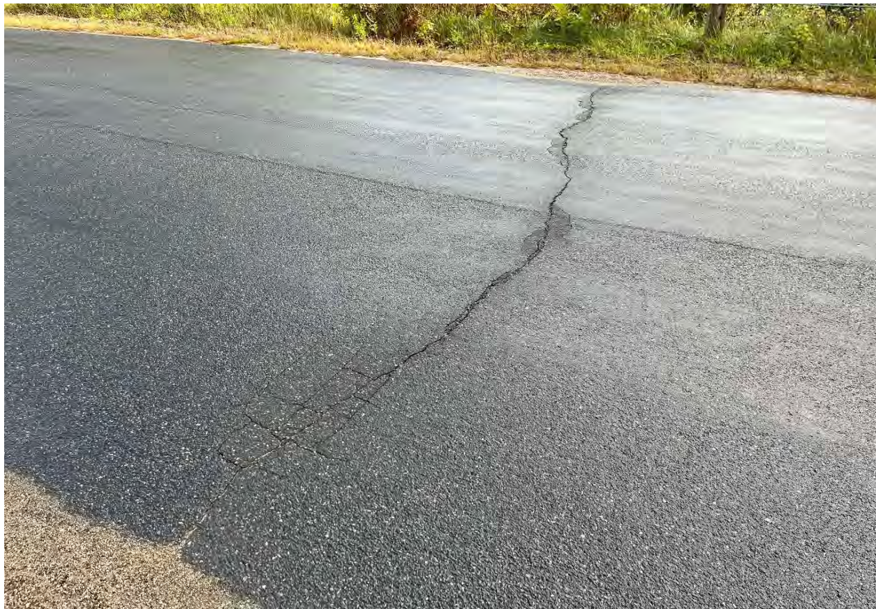
Description of Photo: Transverse crack
