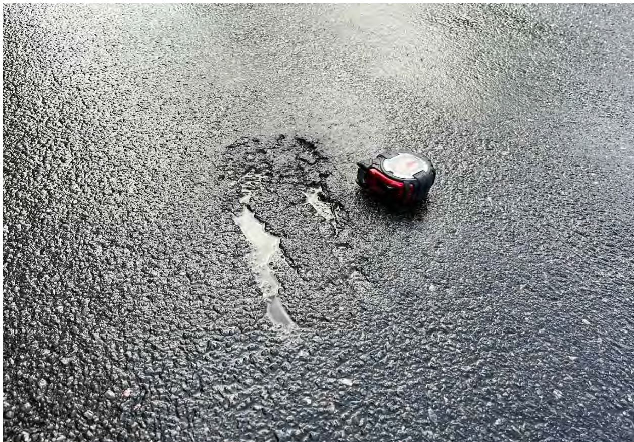
Description of Photo: Isolated severe abrasion
