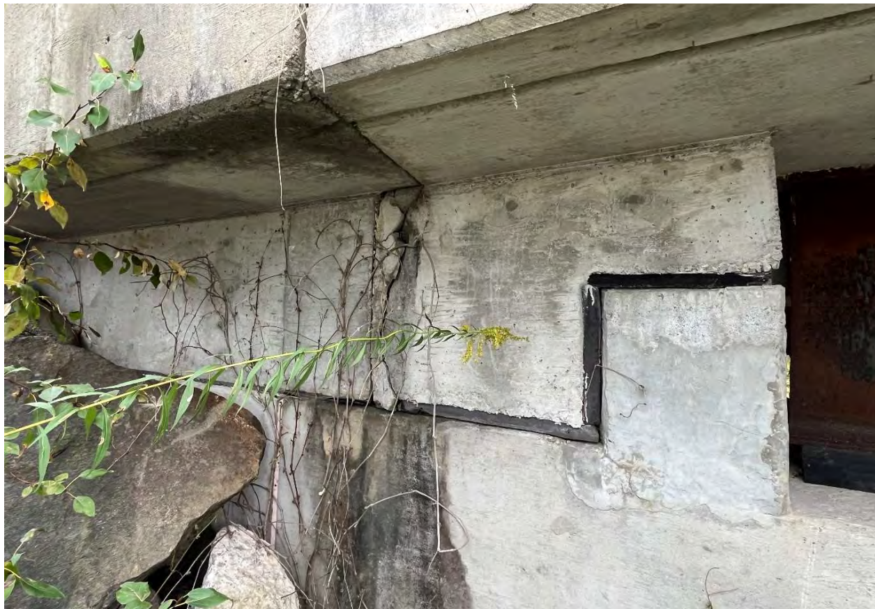
Description of Photo: Isolated delamination
