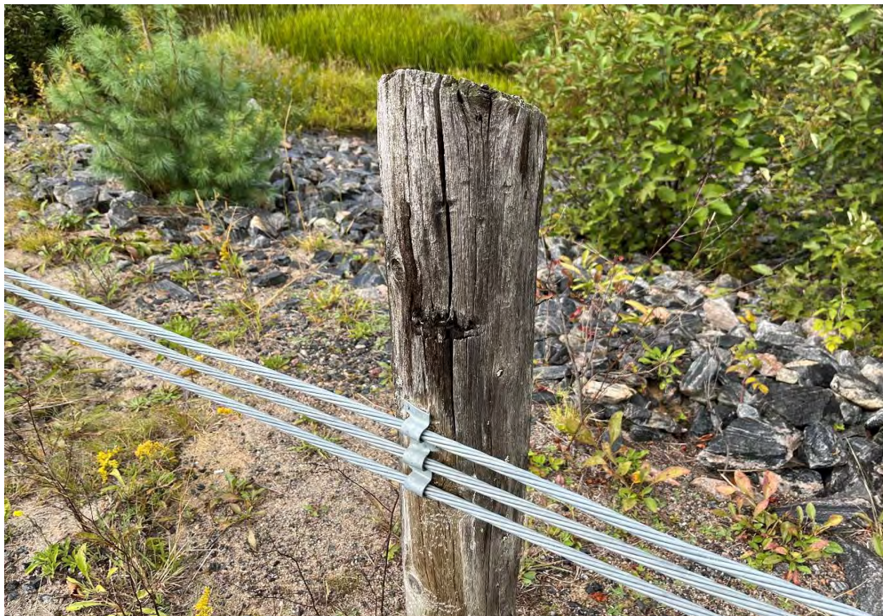
Description of Photo: Post deterioration, typ.
