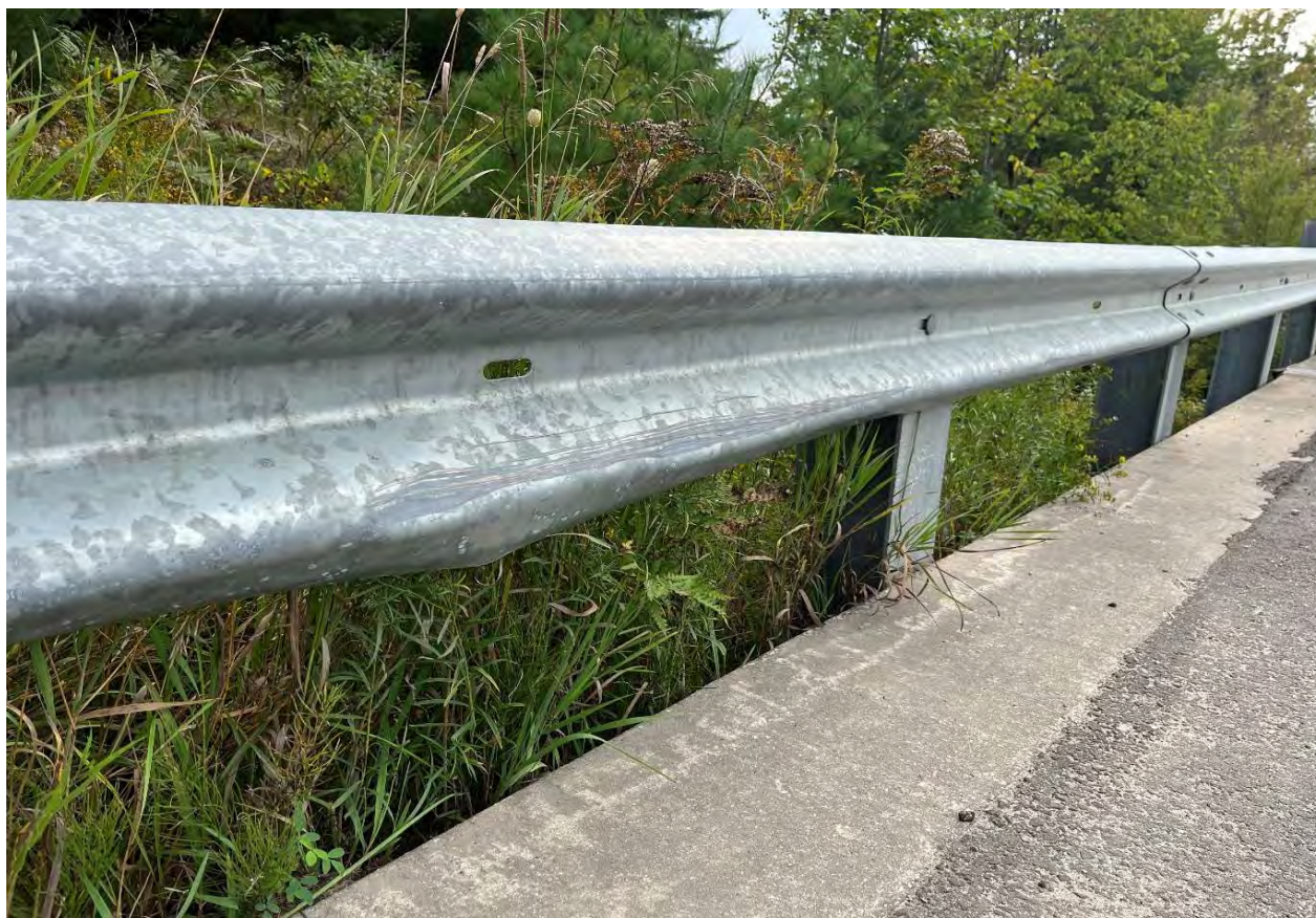
Description of Photo: Isolated deformation, typ.
