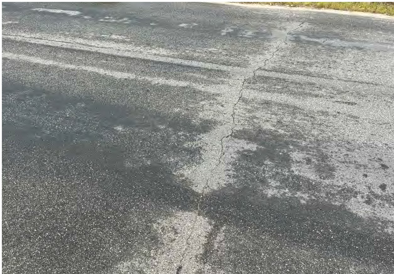
Description of Photo: Transverse crack
