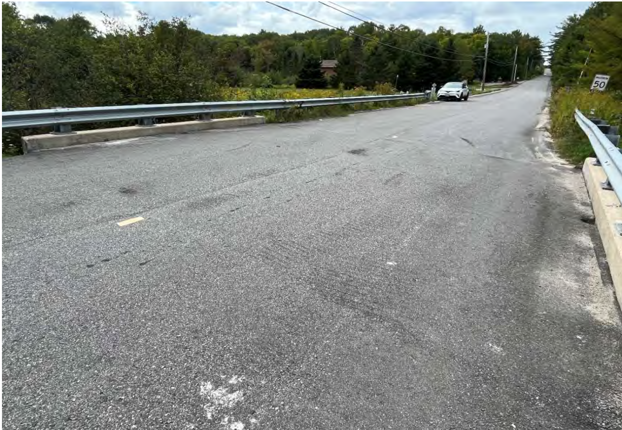
Description of Photo: Asphalt covered concrete deck
