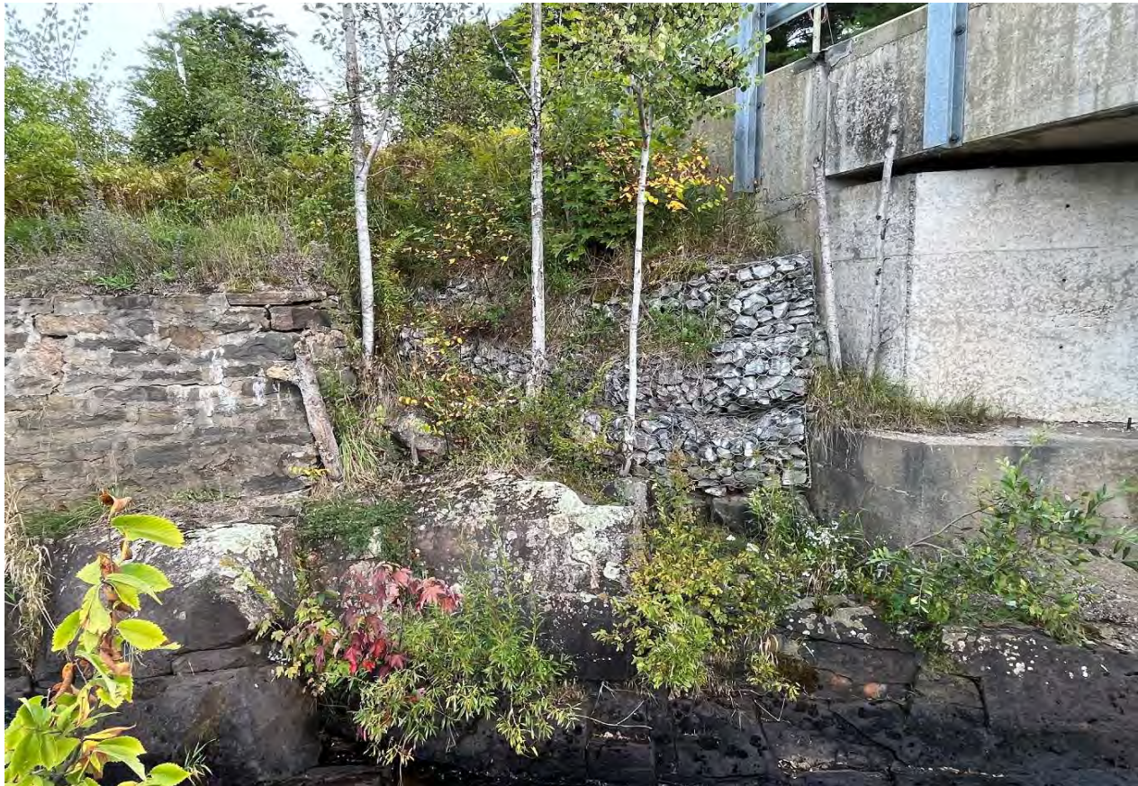
Description of Photo: Northeast gabion retaining wall
