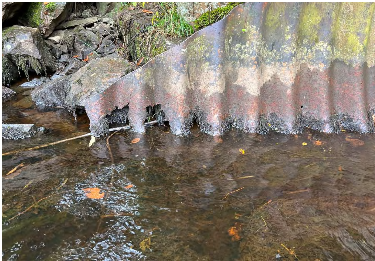
Description of Photo: Section loss at inlet
