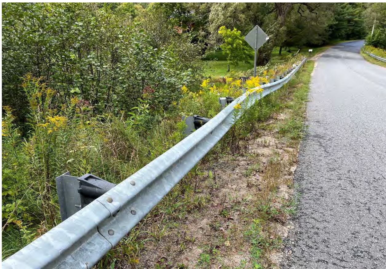
Description of Photo: Approach guide rail - impacted damage
