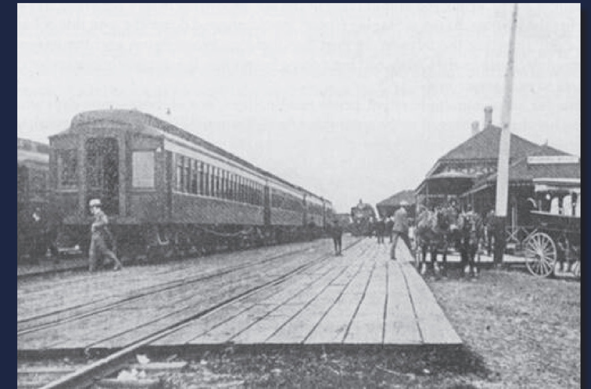
Cockburn strove vigorously to bring a railway to Gravenhurst. His efforts met with success in 1875 when the Northern Railway (later part of the Canadian National system) reached Gravenhurst and the Muskoka Wharf. This led to a boom in lumbering and tourism.
