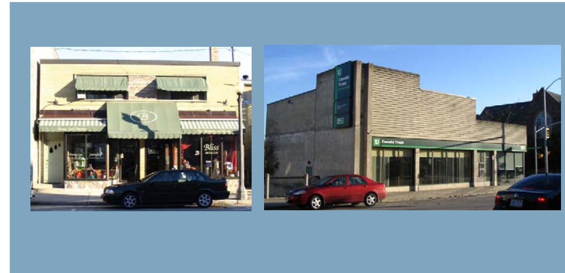
Highest Scoring Image (3.34) Retail, basic brick facade, unifying green retractable awnings, green detailing.
