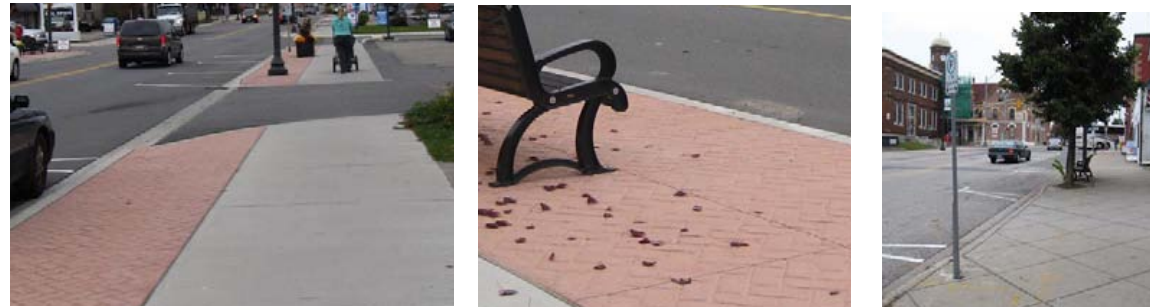
Existing sidewalk pavements in Uptown.
