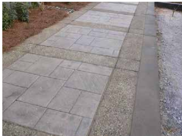
Combination patterned concrete with plain concrete
