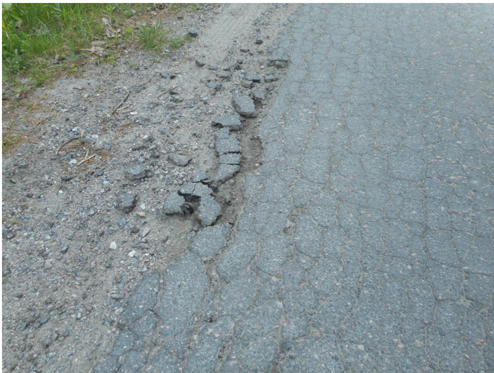
Figure 8: Alligator Cracks and Pavement Edge Breakup on Reay Road (Section 1233)
