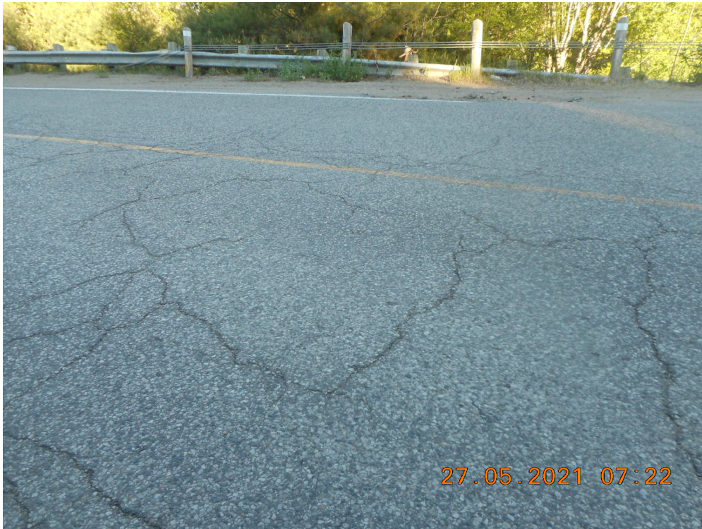
Figure 4: Map Cracks on Sedore Road (Section 1624)
