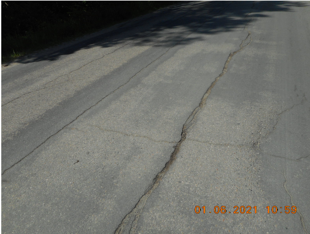
Figure 4: Map Cracks on Sedore Road (Section 1624)
