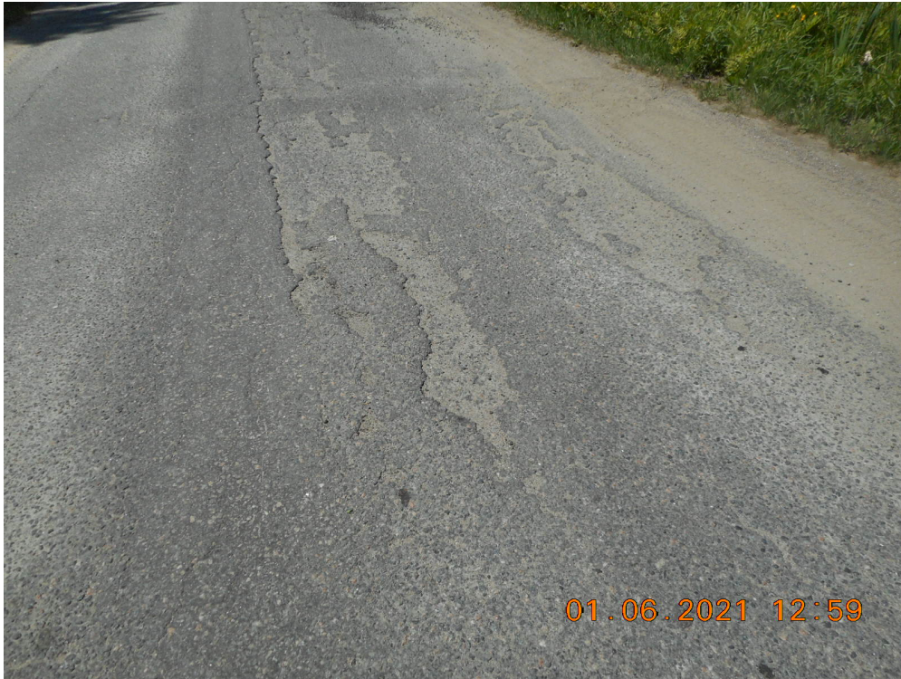
Figure 8: Alligator Cracks and Pavement Edge Breakup on Reay Road (Section 1233)
