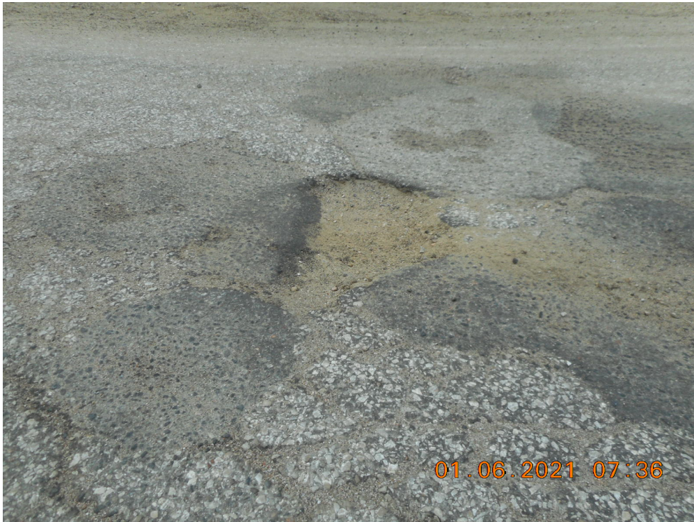
Figure 6: Pothole on Kilworthy Road (Section 1237)
