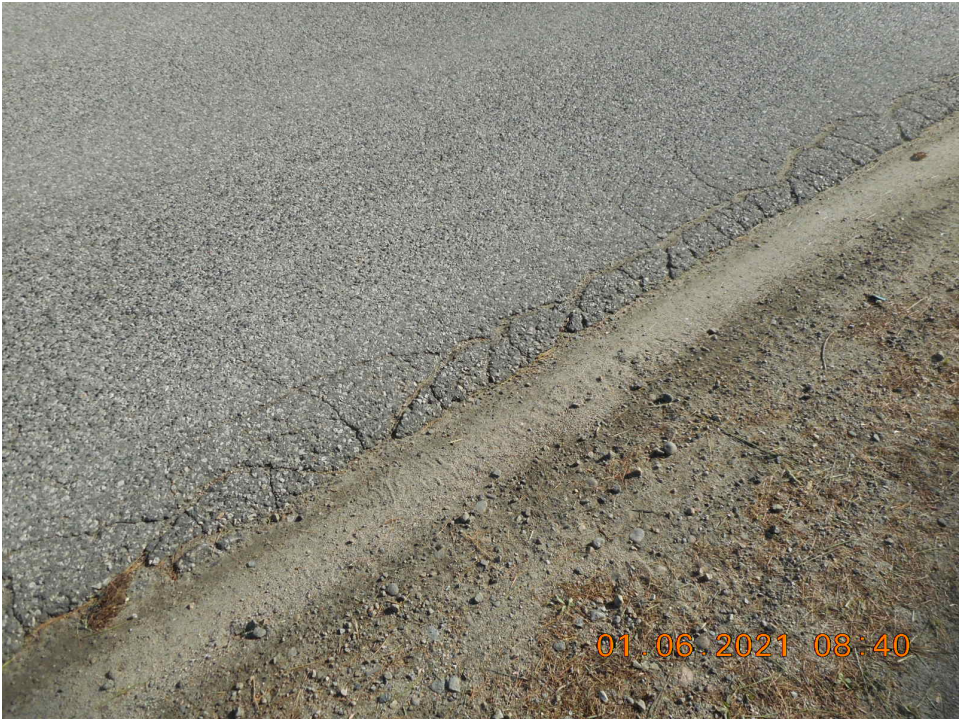
Figure 2: Pavement Edge Cracks on Tryon Drive (Section 1622)
