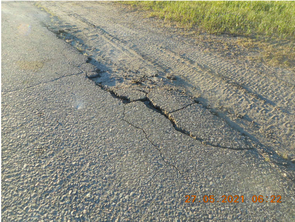
Figure 6: Pothole on Kilworthy Road (Section 1237)
