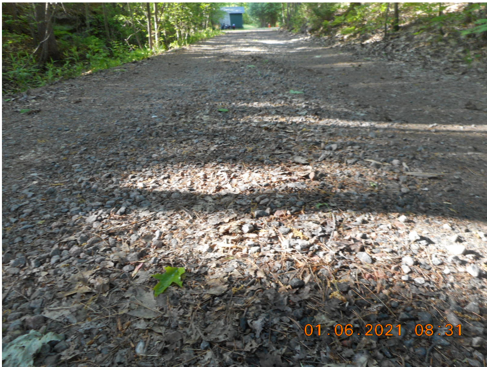
Figure 10: Flat/Reverse Crown on South Bay Road (Section 2038)
