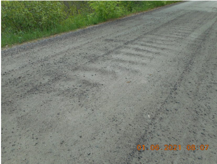
Figure 11: Washboarding on South Kabshe Lake Road (Section 1675)
